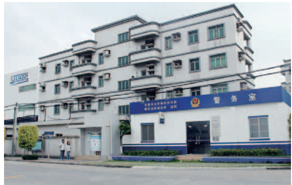
The branch police station adjacent to the GRT building (right) and post office ATM (left)
