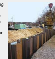
Soil remediation work
