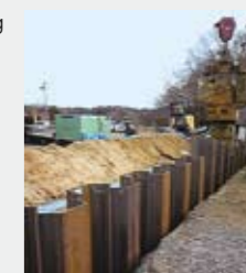
Soil remediation work
