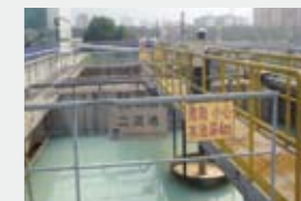
Chemical treatment COD removal facilities
