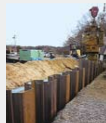
Soil remediation work
