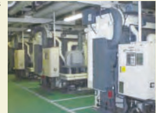
Upgraded absorption refrigeration units
