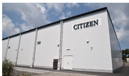
Precision Machining Plant, Karuizawa Headquarters Factory
