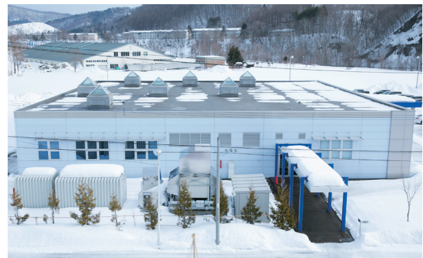
Ambient air cooling and displacement ventilation system
