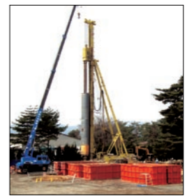
Construction to prevent dispersion of groundwater
