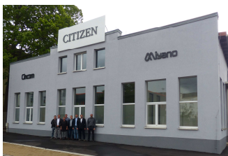
Citizen Machinery Europe GmbH Technical Center East
